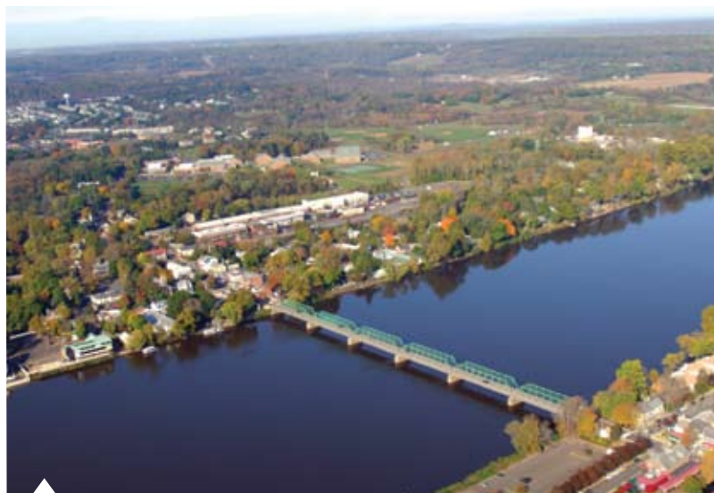
NEW HOPE/LAMBERTVILLE BRIDGE
